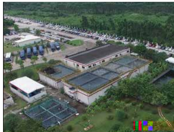
Wuyang-Honda Motorcycle's Wastewater Treatment Project
