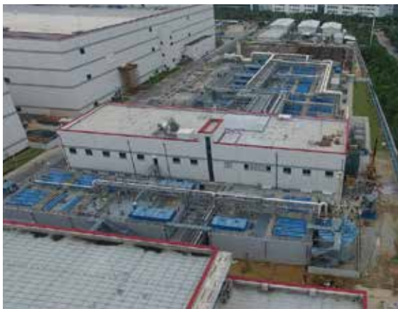
LG Display's Wastewater Treatment Project
